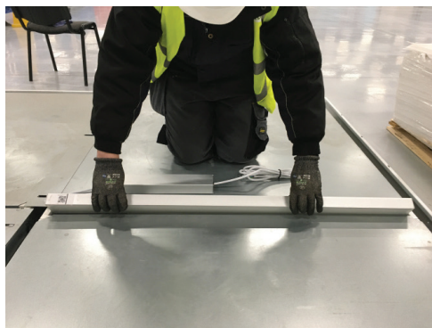
Separate gear enclosure and insert Luminaire into noggin
