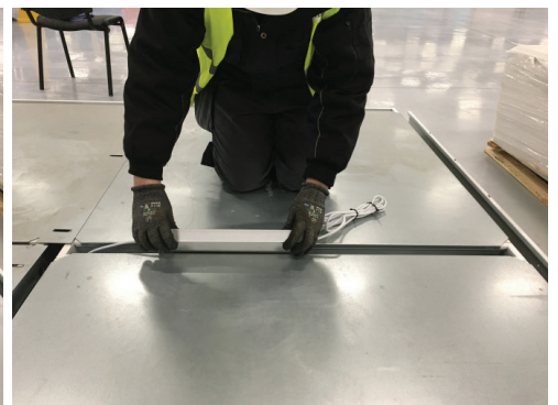
Carefully insert gear enclosure into noggin
