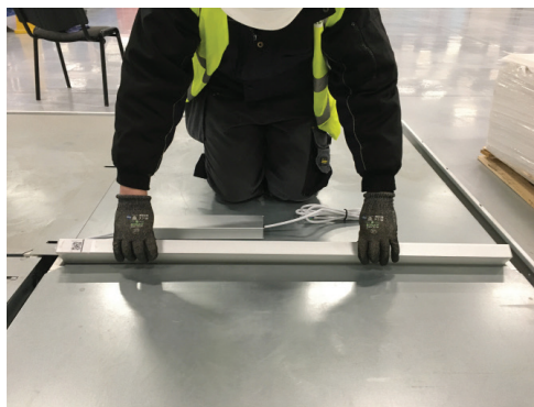
Separate gear enclosure and insert Luminaire into noggin
