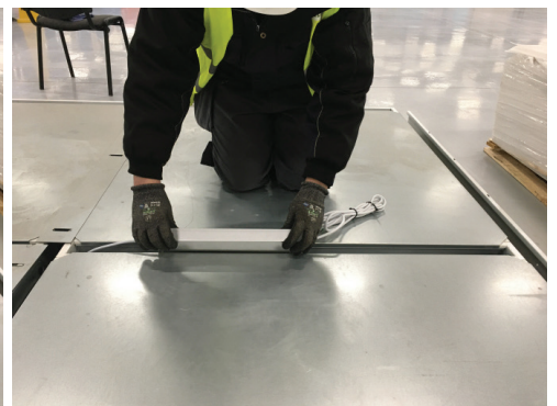
Carefully insert gear enclosure into noggin
